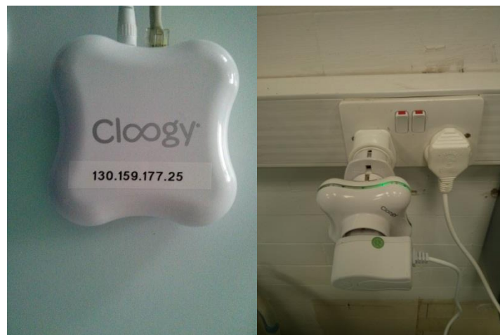
Figure 7 Hub lab setup battery capacity test
