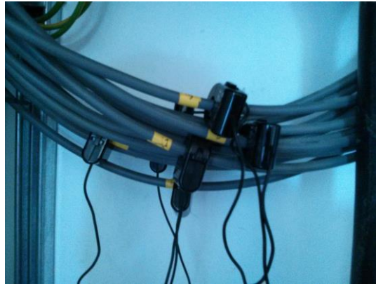
Figure 6 AlertMe incomer clamps on Soillse incomers
